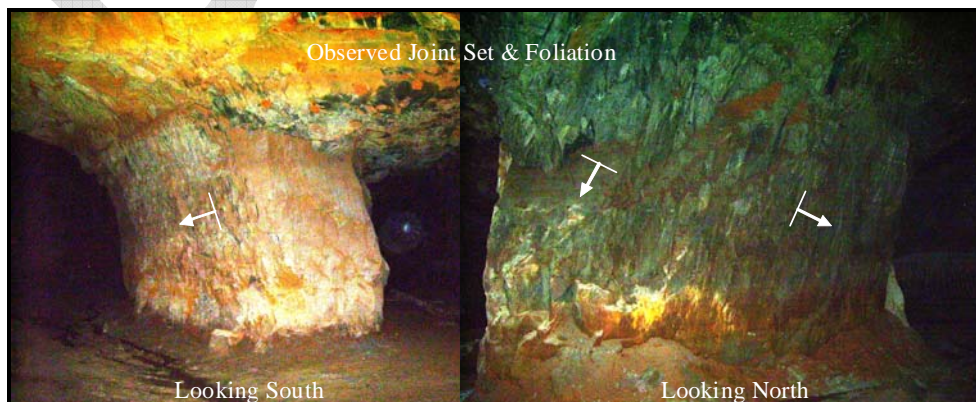
Figure 8.3 Pillar (Between Ramp and North-South Exploration Drift)
